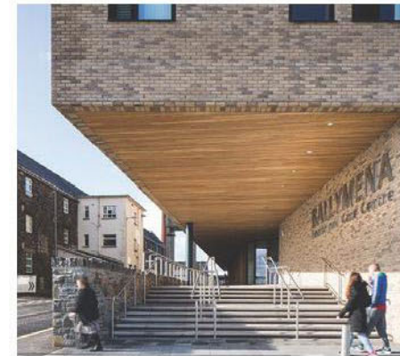
TIMBER SOFFIT TO TERRACES + PODIUM
